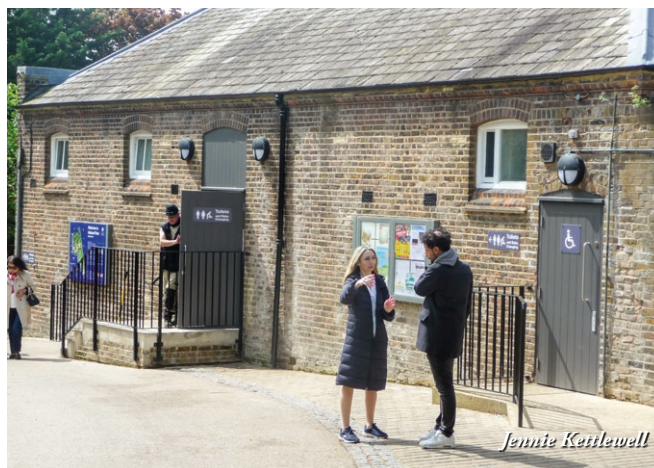
New toilets, with main door on left and radar key access door on right
