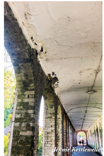
Damage to ceiling above marouflages.
