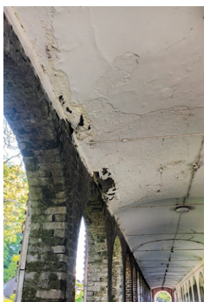
Water-damaged roof over paintings.
